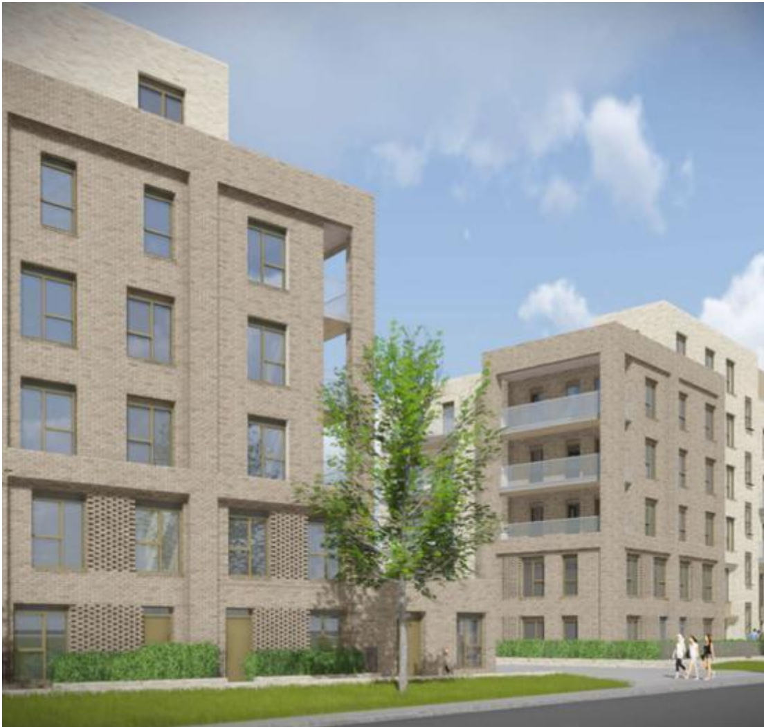
View along Winchelsea Road - Corner elements of Blocks C and B
